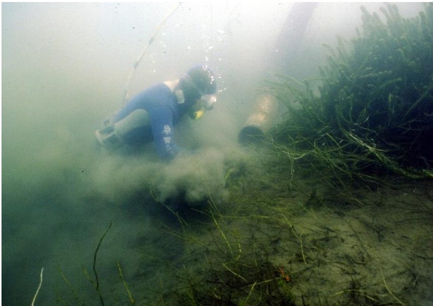
Figure 18 Diver directed suction dredging in Lake Wanaka (Photo: J. Clayton, NIWA).
