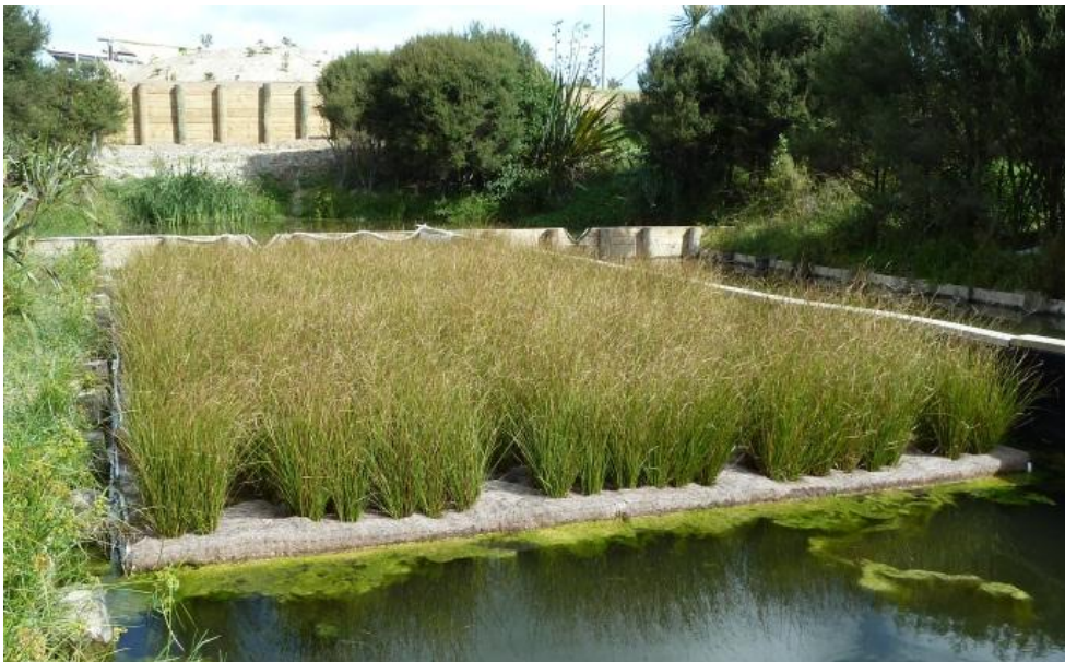
Figure 14 Floating island in place on motorway stormwater treatment pond in Silverdale, North Auckland. (Photo: C. Tanner, NIWA).
