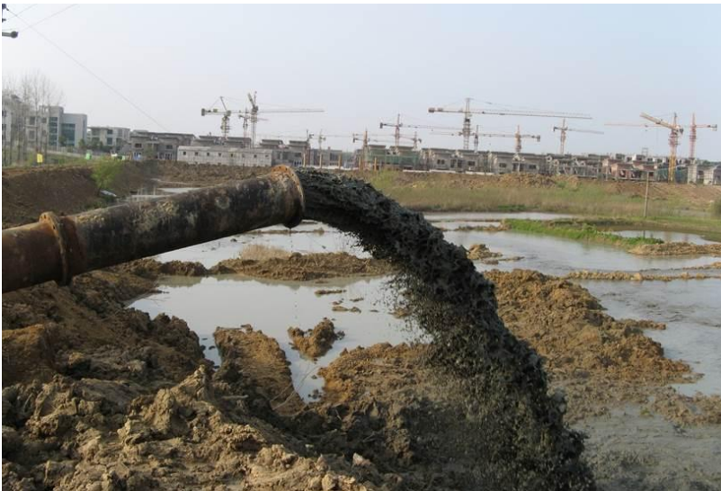
Figure 21 Dredged spoil pumped from a dredging operation on a lake on the Yangtze River delta (China).
