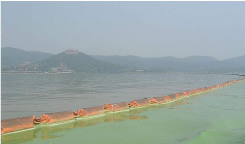
Figure 23 Outer wave-attenuation barrier installed to protect a water treatment plant intake in Lake Taihu, China (Photo: Liancong Luo)
