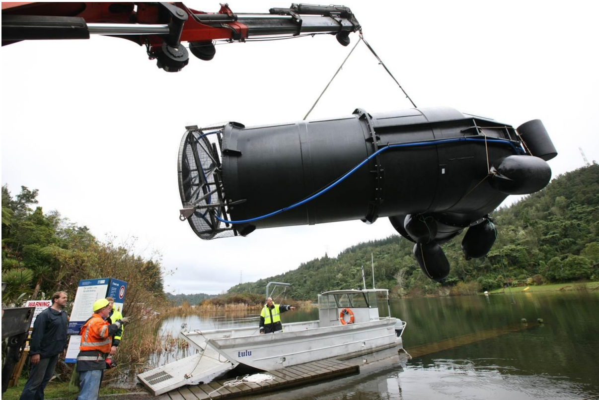
Figure 22 Part of an artificial destratifier being installed at Lake Rotoehu, Bay of Plenty. Note screen at bottom intake (left hand side).
