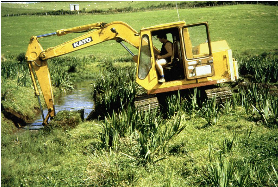
Figure 16 Digger removal of yellow flag from a drainage system (Photo: R. Wells, NIWA).
