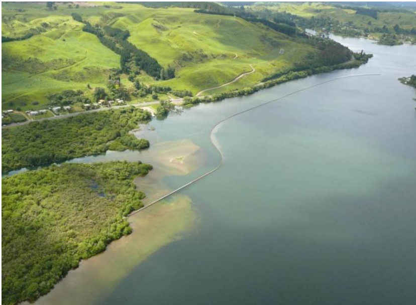
Figure 24 Ohau diversion wall, Lake Rotoiti. Ohau channel enters on left hand side and is directed towards the Kaituna River outlet towards top of photo (Photo: Andy Bruere).
