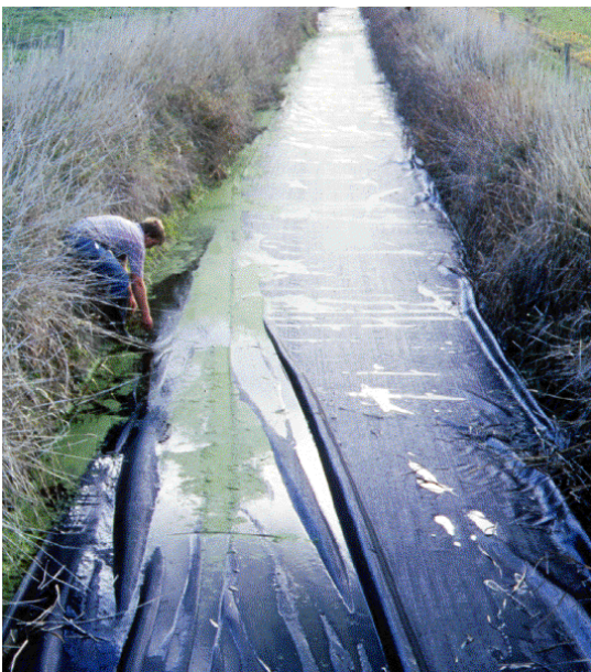
Figure 13 Surface cover fitted over a ditch system to control aquatic vegetation (Photo: R. Wells, NIWA).
